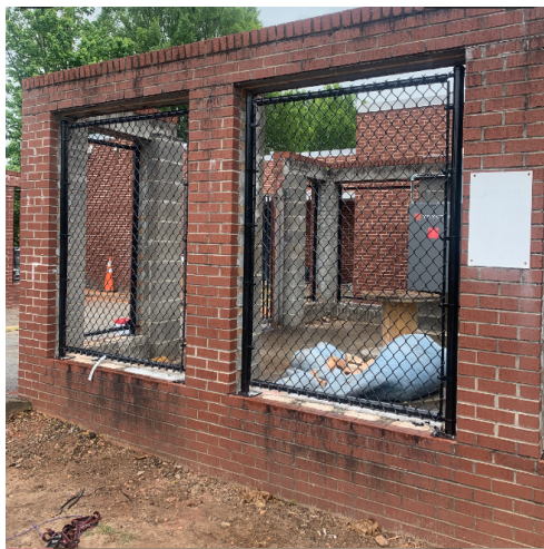
Installed fencing for generator enclosure.
