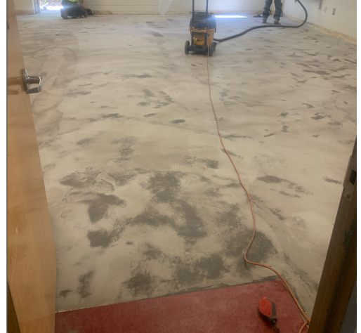
Started floor prep and working on install of VCT of the 1st floor classrooms.
