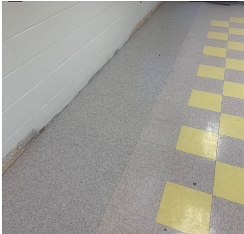
Started install of VCT at 2nd and 3rd floor classrooms.
