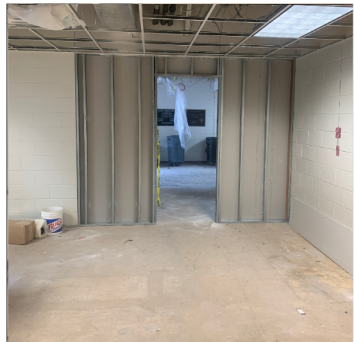
Temporary wall has been framed up in the main entrance/ administration area.
